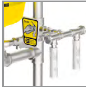
Note: External drain temperature sensing valves
